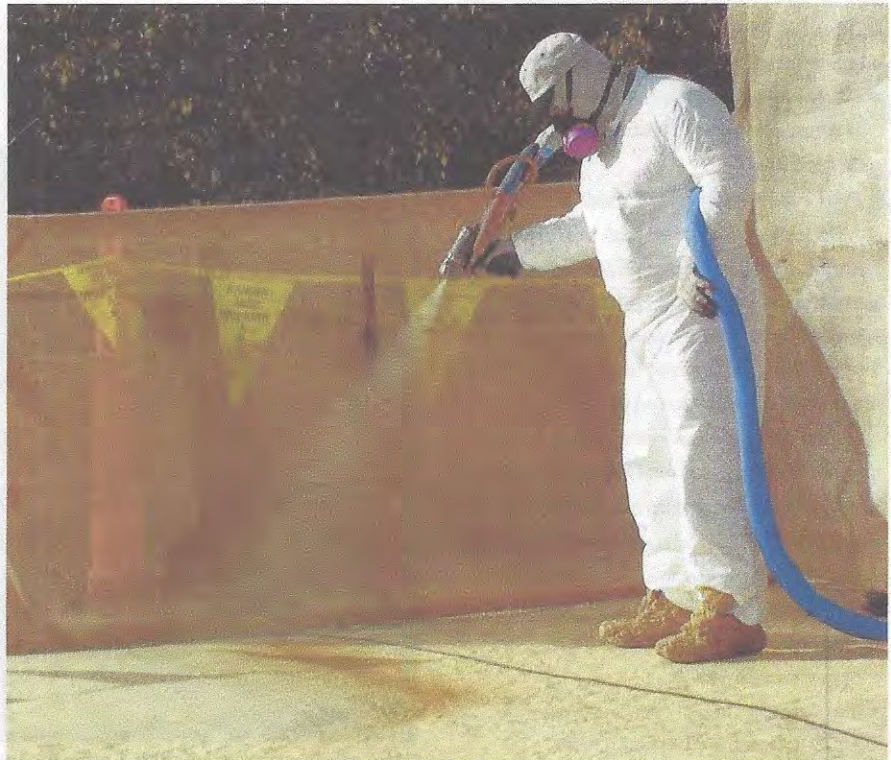
SPF can be installed on wood, concrete, metal, asphalt, foam sheathing and more. But the substrate must be clean and dry. Photo courtesy of Honeywell.
