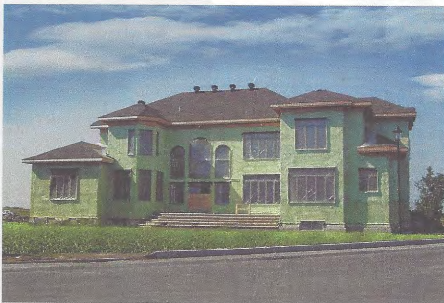
Spray techniques for closed-cell SPF differ from those for open cell. The spray technique can affect the quality of the foam application. Photo courtesy of Demilec.
