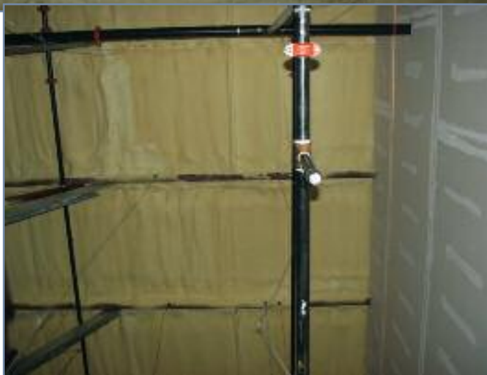
Photos 3 and 4 – Here, ccSPF is installed to the interior of a metal building without studs. This type of application has an added benefit of reducing thermal bridging through the metal beams and columns.
