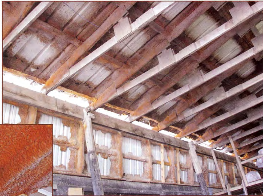
Figure 5 – Old metal secured with ccSPF.
