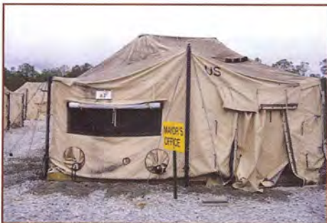
Photo 16 – Example before application of ccSPF.
