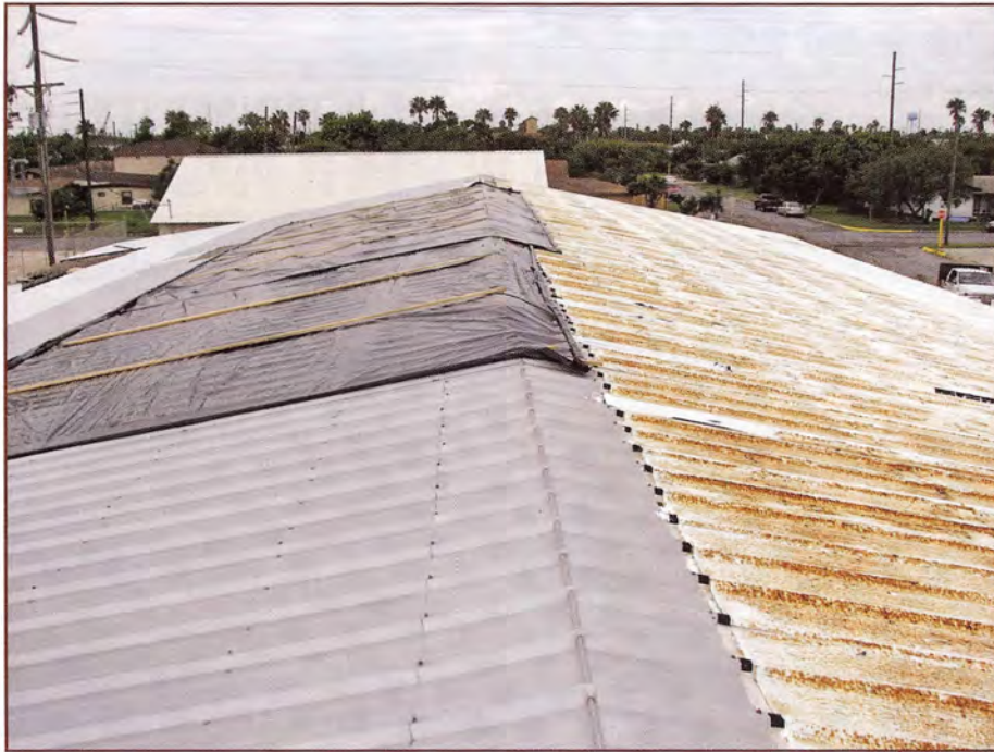
Figures 3 (left) and 4 (below) – Half of the roof blew off of White’s Lumber during Hurricane Dolly.
