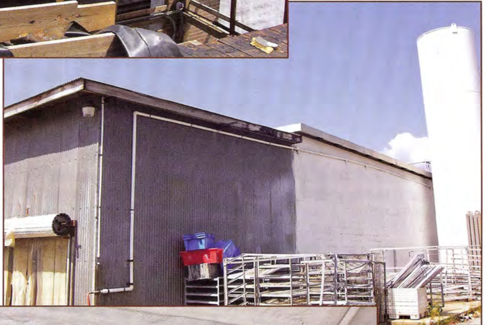
Figure 10 – The metal building below was connected to the structure shown in Figure 9 and was insulated with ccSPF. It received no damage during Hurricane Katrina.
