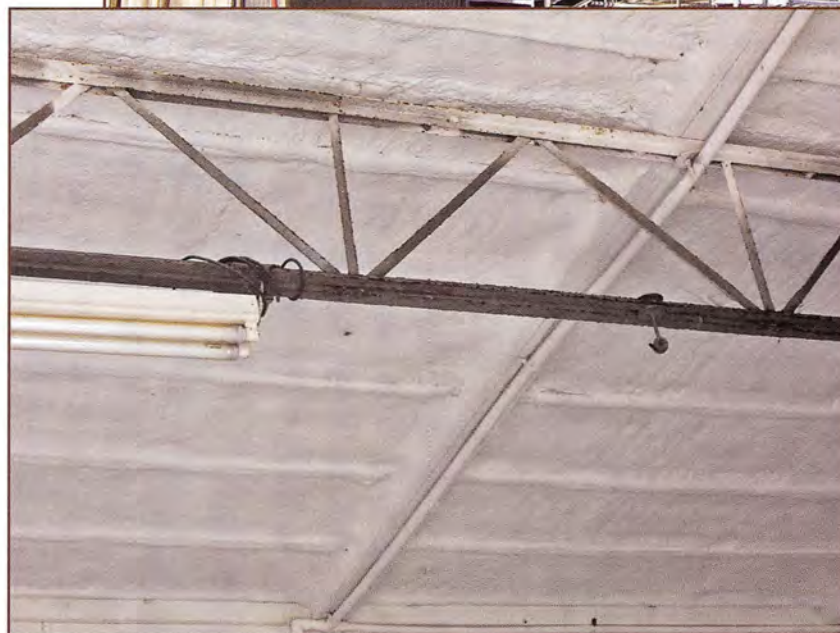
Figure 11 – Foam sprayed against metal roof decking and corrugated metal wall panels.
