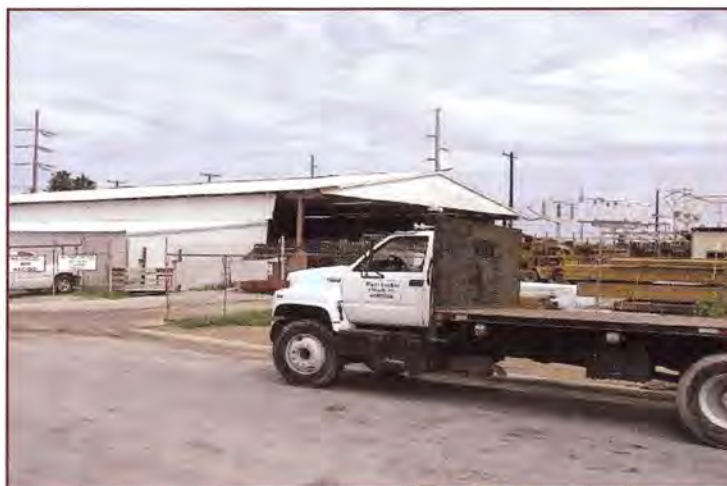
Figure 2 – The author installed the old metal roof on this building in 1980. A new metal roof was installed in 2008 on the right side of the building.
